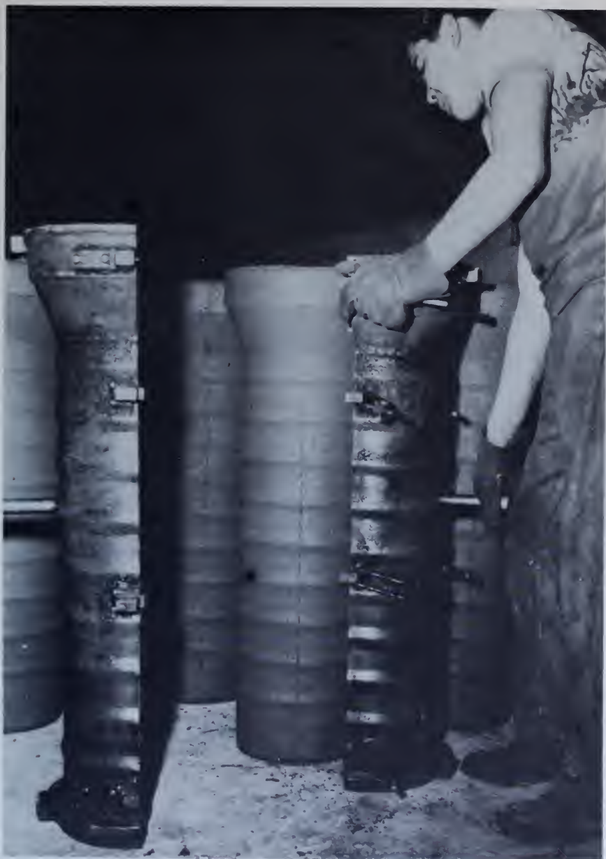
Figure 168.—Form removal from unreinforced packerhead pipe immediately after placement. PX-D-34072.
